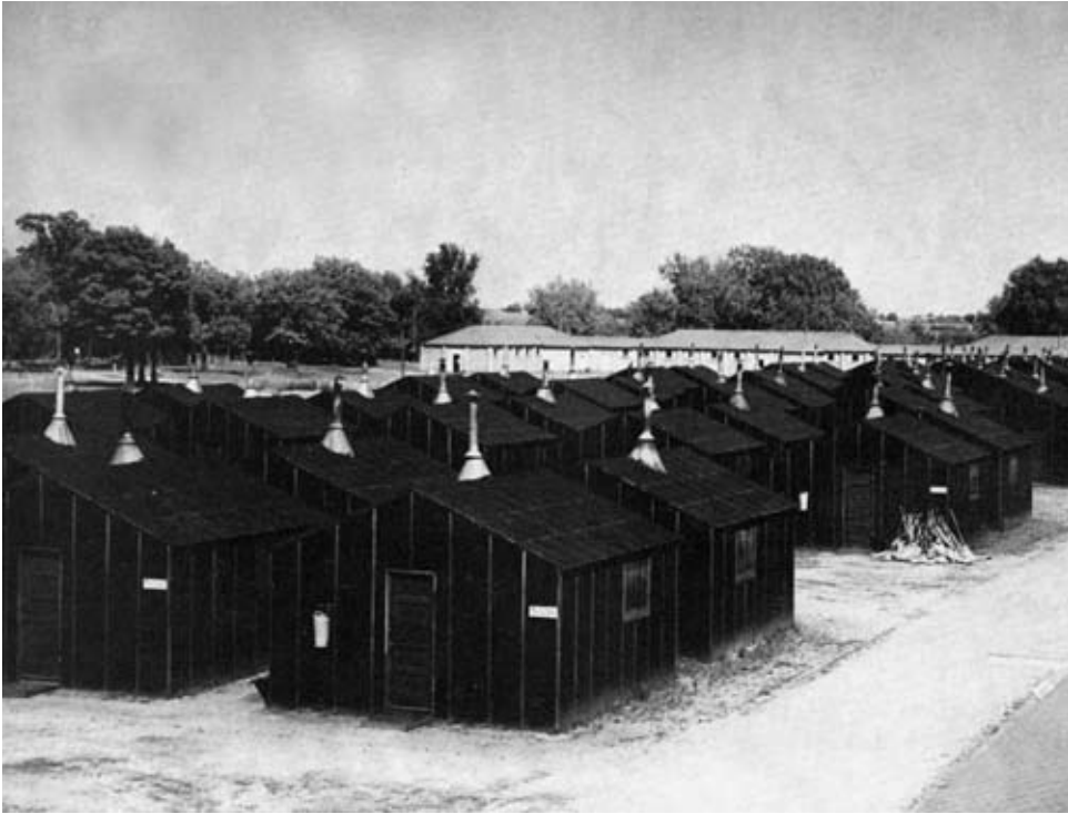
Temporary barracks known as the Turkey Farm
